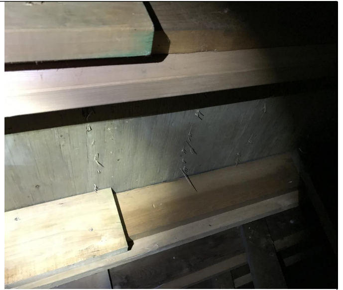
Photo 2 – Roof Rafter Reinforcement
