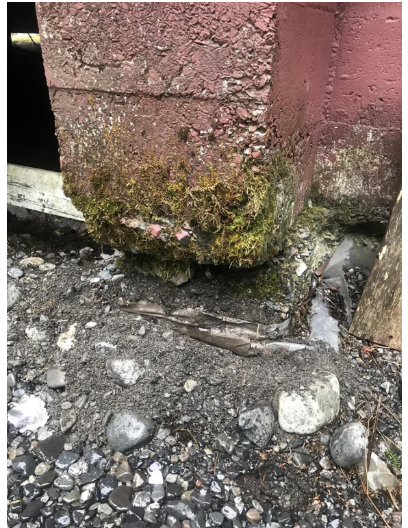
Photo 6 – Concrete Pier at Grade
