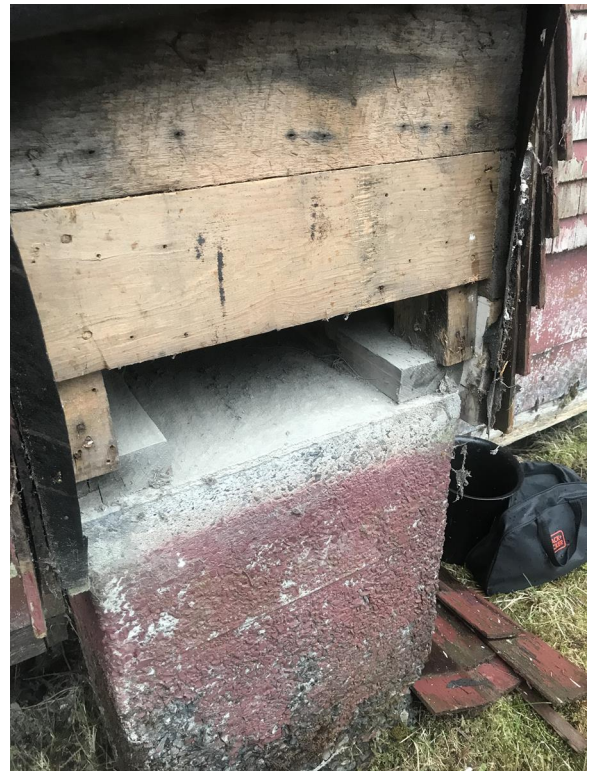
Photo 4 – Exterior Pilaster Wood Framing
